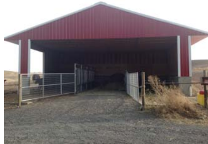
Off-stream heavy use area includes fencing, off-stream water, shelter, access road, and waste storage facility.
