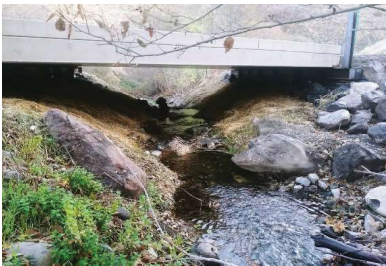
New bridge and instream habitat improvement replace barrier culvert and allow passage for adult and juvenile Snake River steelhead. Photo credit: Lovina Englund
