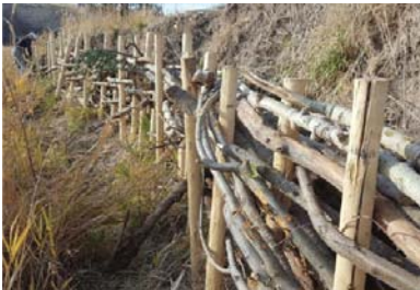
As a foundation for sediment deposits, woody debris is installed behind this bank stabilization project. Photo by Emily Novack
